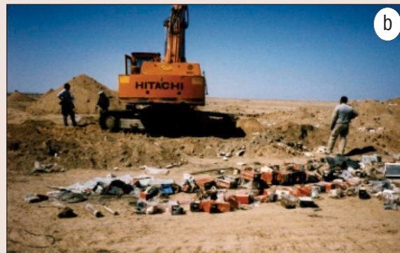
Figure 7. (a) Two-frequency electromagnetic data over a 7-acre nuclear burial site. The grid size is 100 ft by 100 ft. The burial pits are indicated by red anomalies. Red-yellow bands in the high-frequency quadrature data were identified as dry streambeds. (b) Excavation based on data shown in Figure 7a. Most items excavated at this site, carefully packaged on wooden pallets, contained various nuclear-related parts and instruments.
